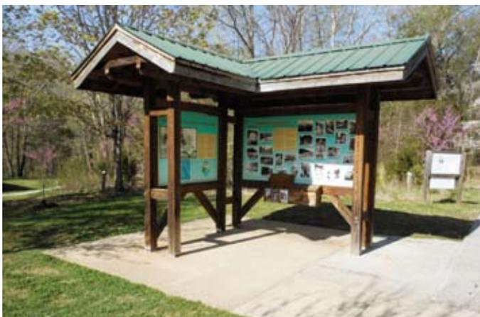
Figure 7: Nine Year Old HVFA PCC Slab without a Crack 4/20/14
