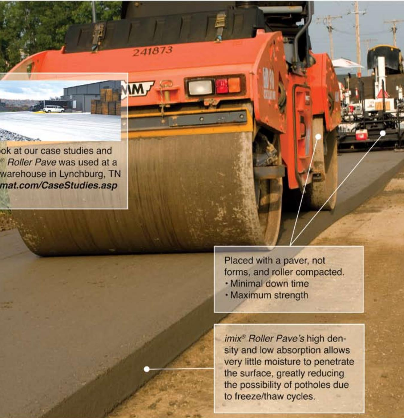
Placed with a paver, not forms, and roller compacted.
