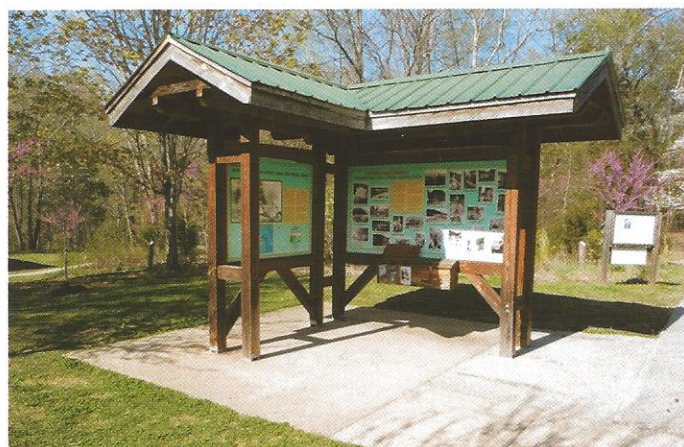
Figure 7: Nine Year Old HVFA PCC Slab without a Crack 4/20/14
