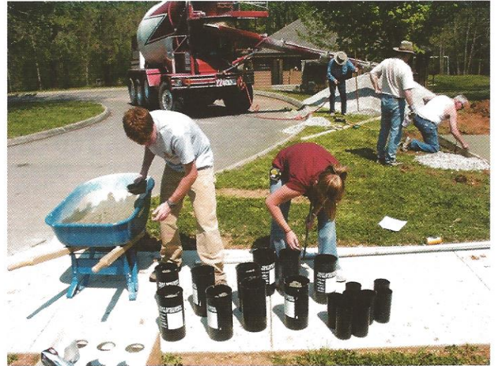
Figure 4: Making Test Cylinders, Finishing and Cleaning Up
