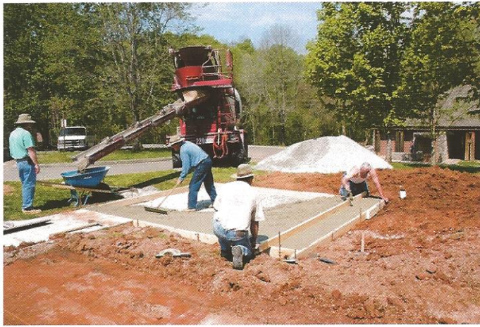
Figure 3: Close Up Showing Grading, Screeding and PCC Sampling
